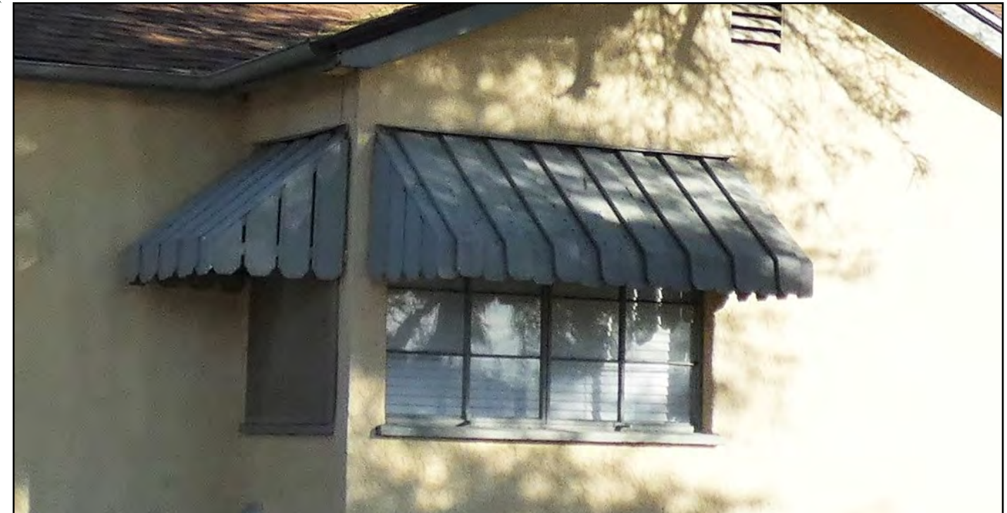
Image 27: Recommend retention of early wood awnings.
