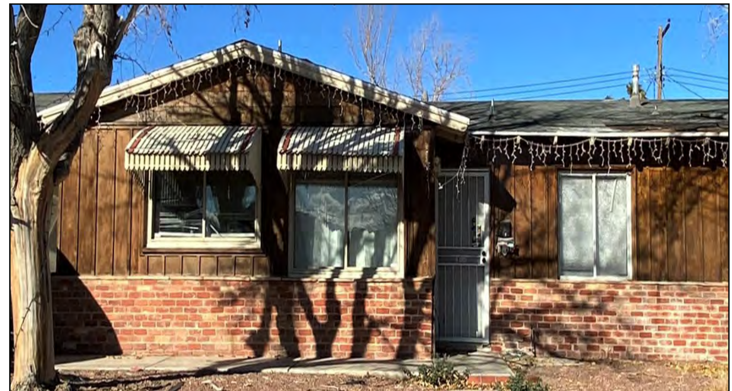
Image 23: Example of typical security door at front entry.
