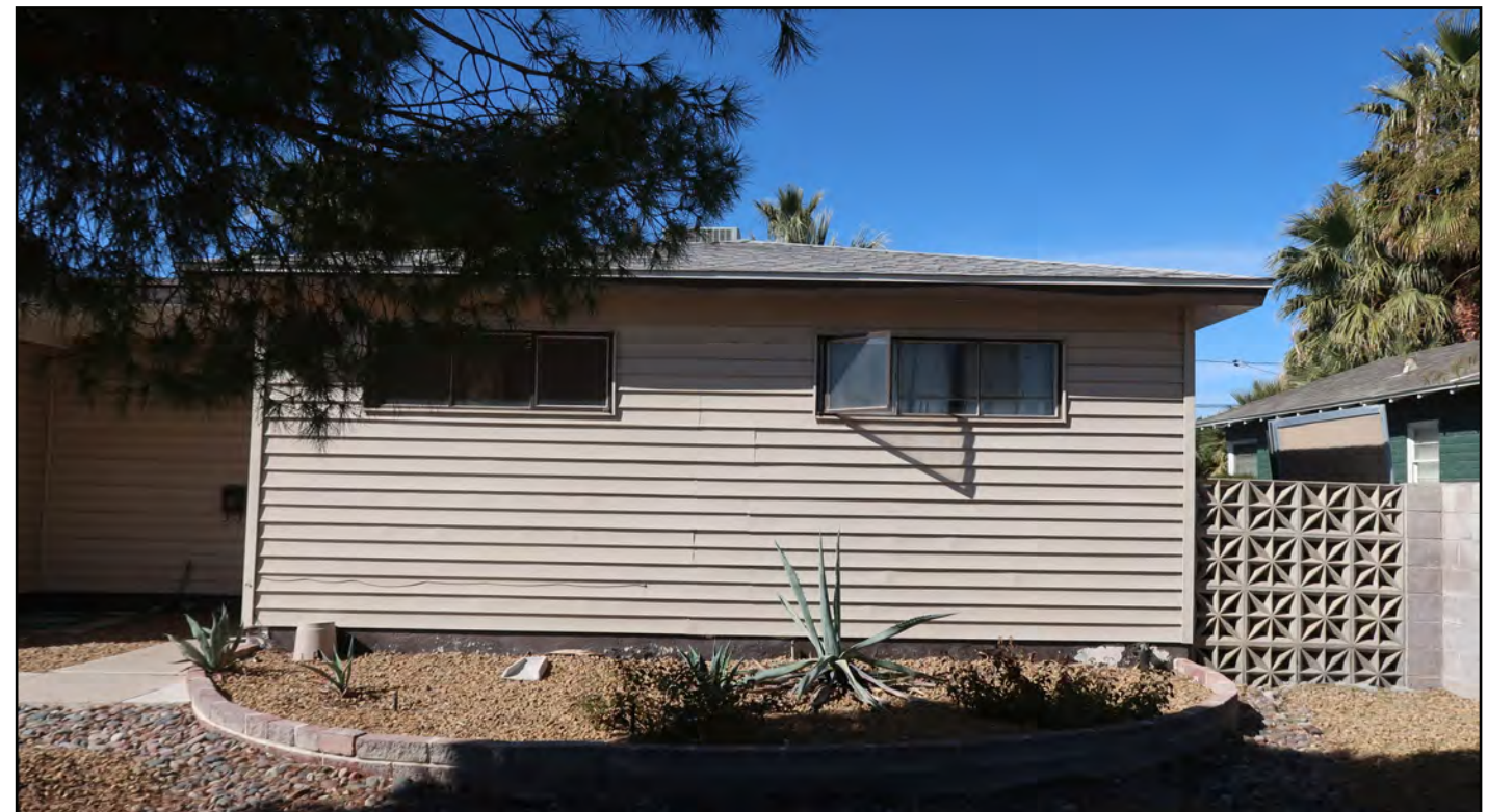
Image 21: Example of vinyl siding.
