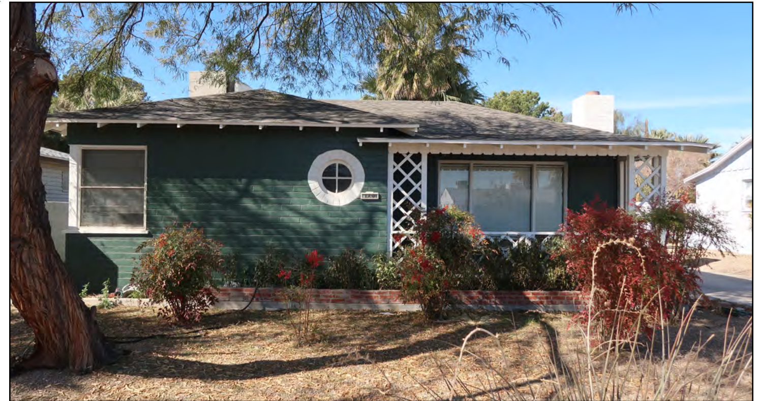
Image 11: Recommend retaining exterior materials, window openings, and exterior detailing at covered porch.
