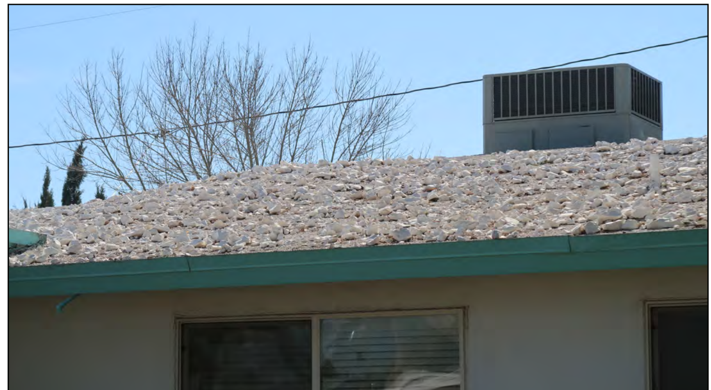
Image 5: Recommend retention of historic rock roof.
