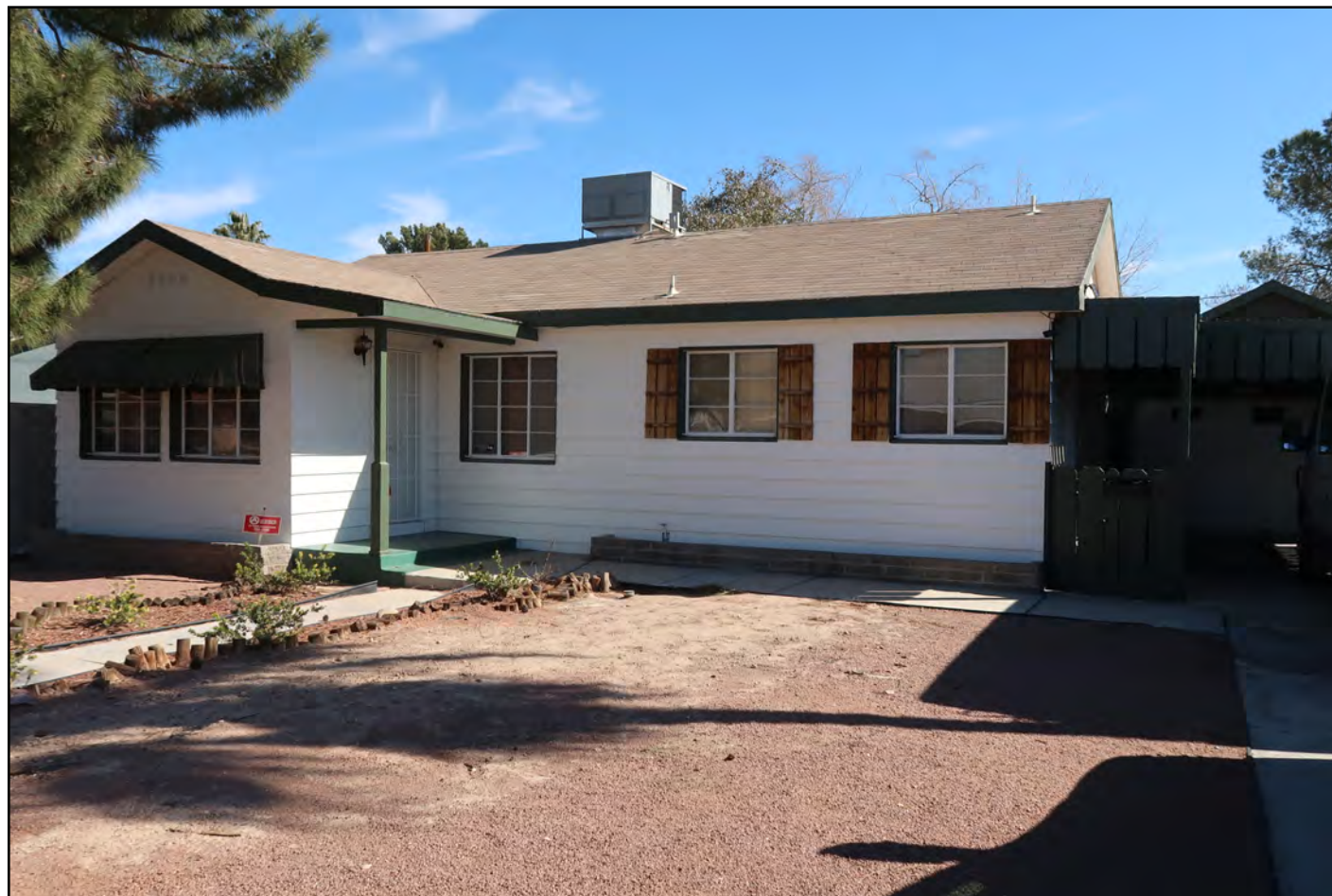
Image 10: Recommended example of in-kind replacement of windows.
