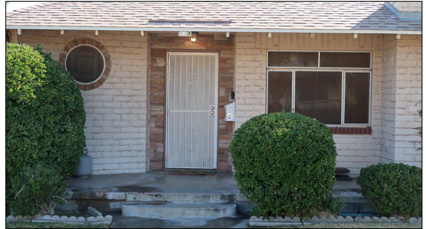
Figure 1: Recommended removable window covers with appropriate light transmittance that follow the shape of the windows.
