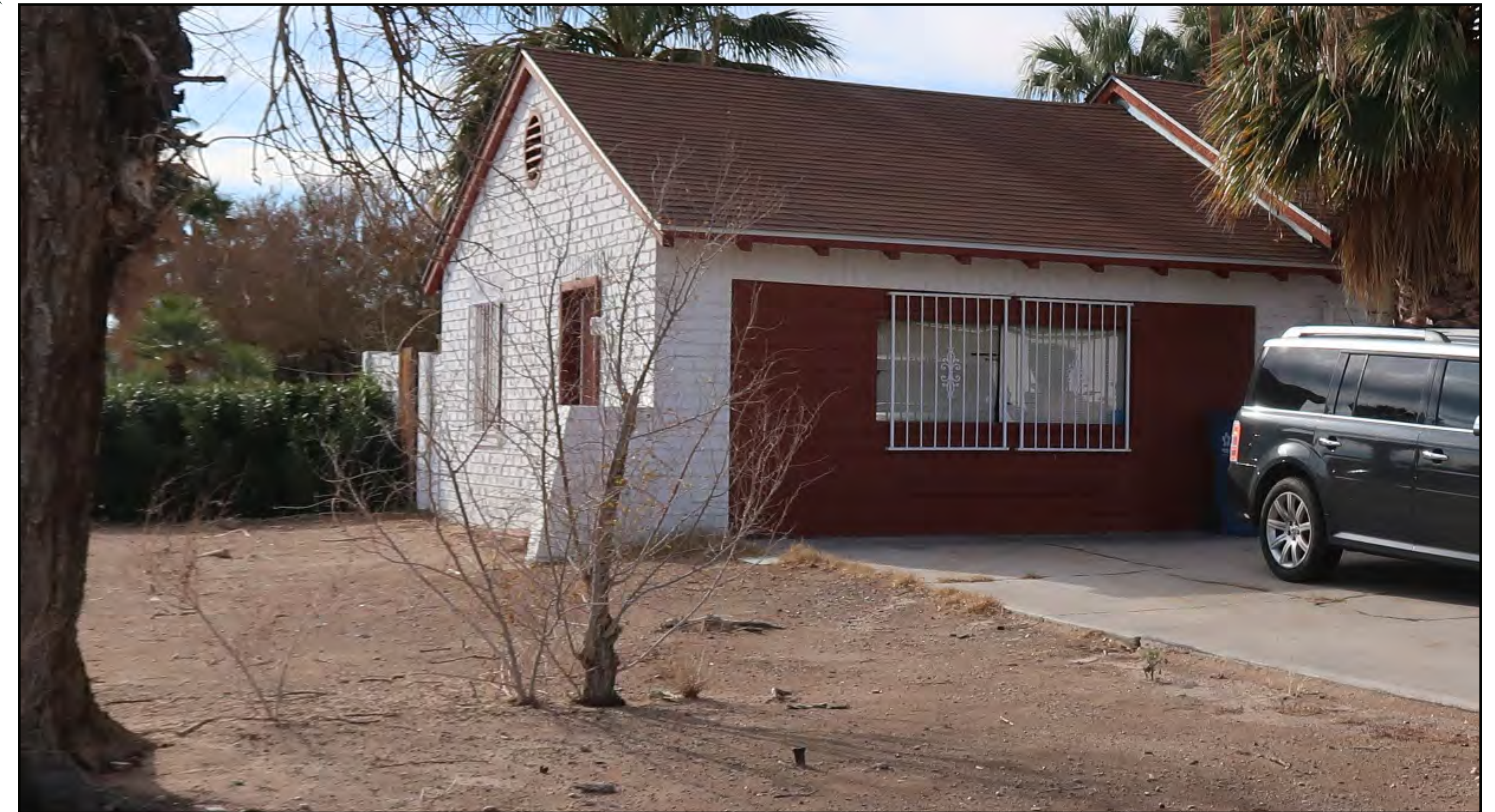
Image 15: Recommended garage/casita conversion. Note a reveal remains where the garage door was replaced.
