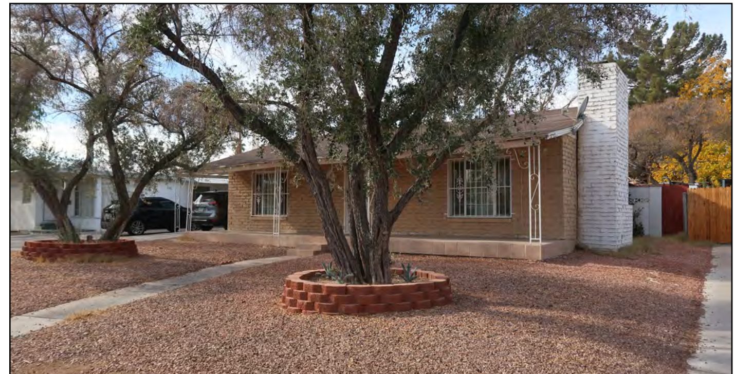
Image 23: Recommended example of altered landscaping that retains mature trees.
