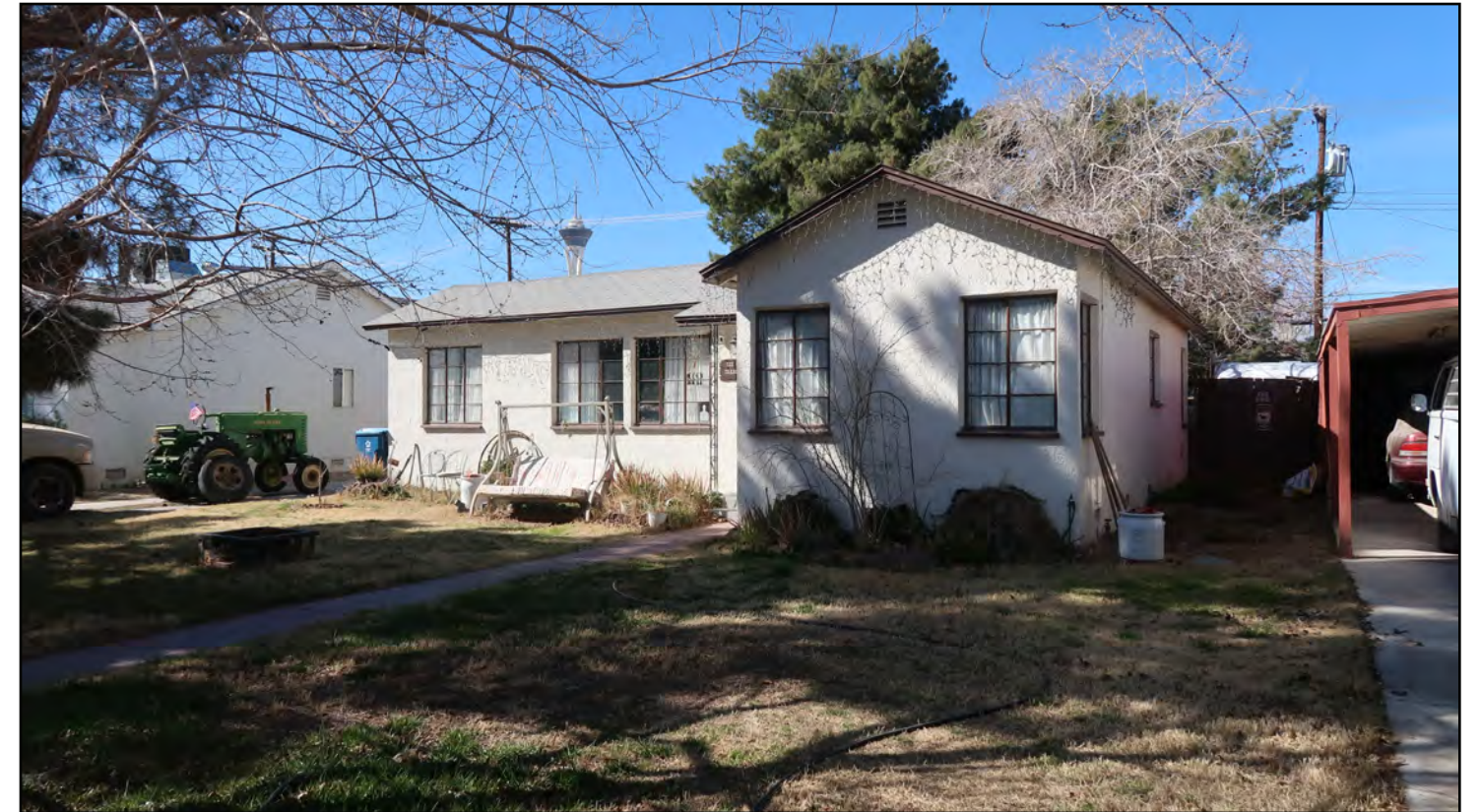
Image 9: Recommend retaining historic windows whenever possible.
